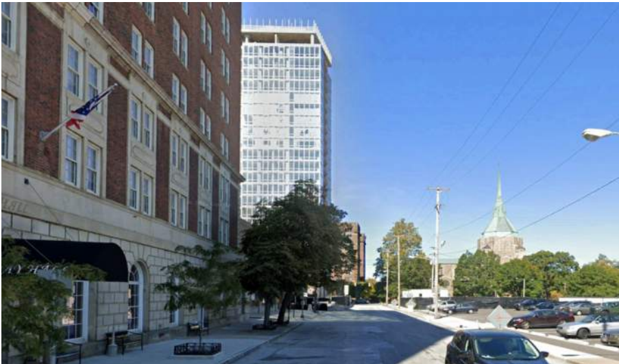
6 - LOOKING NORTH ON STOKES BOULEVARD
